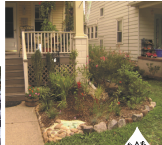
Downspout disconnection with rain garden example
